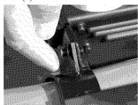
Once all bolts have been installed, tighten all nuts using allen wrench and socket on both bolts and nuts.
